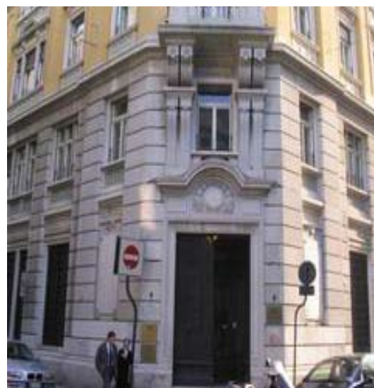
BUILDING OF THE HEADQUARTERS OF THE CEI-ES IN TRIESTE
