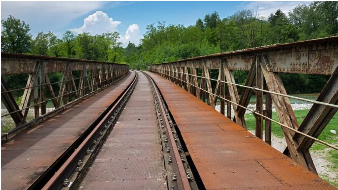
Figure 13: Figures old railway connection and infrastructure on Sacile - Pinzano railway line
